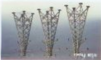
97. Tower crane 96. Tower crane 95. Tower crane
