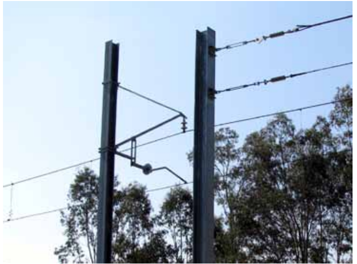
Example of a Fixed Termination Mast.
