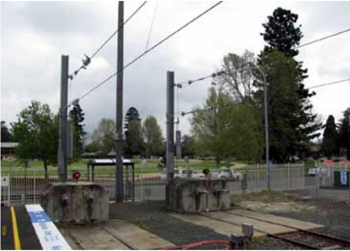
Example of a Termination Spanner.
