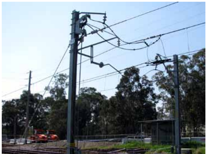
Example of a Feeder Mast.
