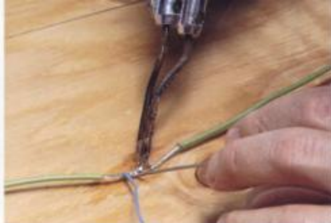
This simple Tee splice connects wires under a layout.
